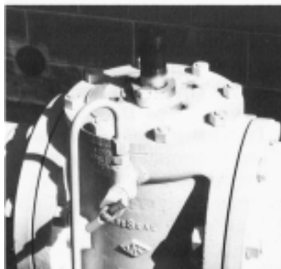
VALVE WITH OPERATOR REMOVED
