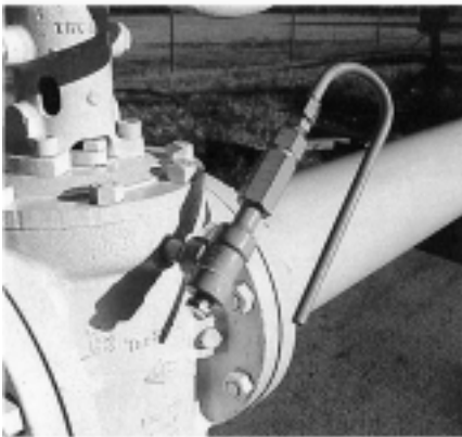
THERMAL RELIEF TO ATMOSPHERE (TRA)
