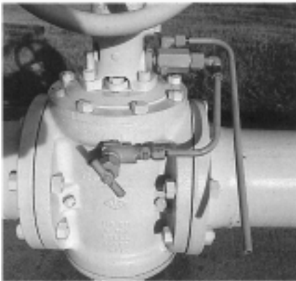
AUTOMATIC BLEED VALVE (ABV)
