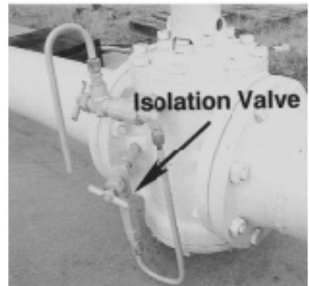
MANUAL BLEED WITH THERMAL RELIEF (MTR)
