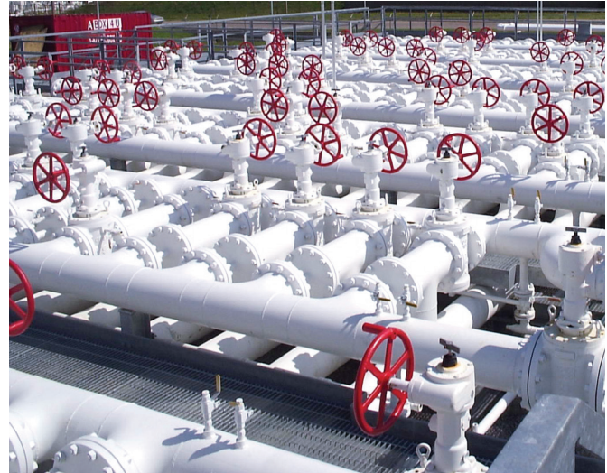
Contamination is avoided in multi-product manifolds.
