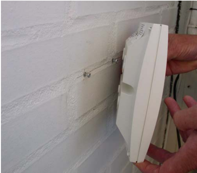
Figure 12 Wireless Server 600v3 Wall Mounting
