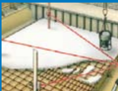
Levelling Slabs
