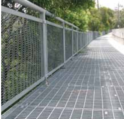
DM3032 – Balustrade infill panels
