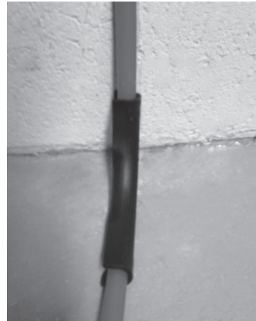
Use the Warmup Pipe Bend Support where it enters the floor.
