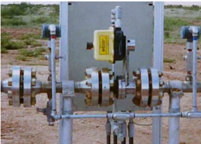
MOV inline/axial choke electrically actuated.
