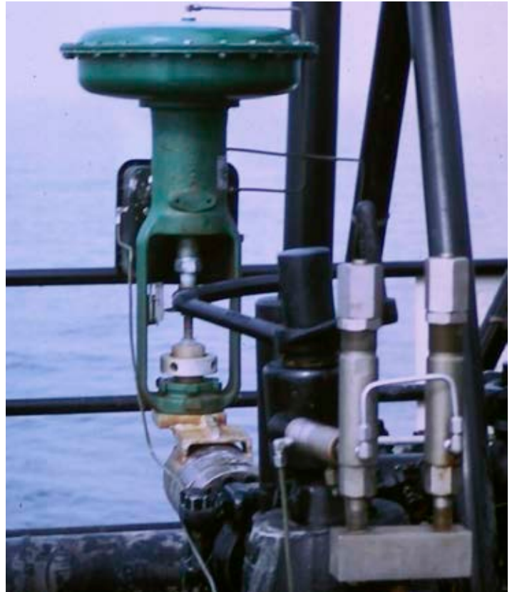
Pneumatic diaphragm actuated MOV choke.
