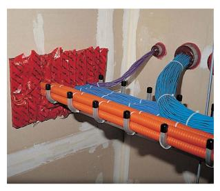
Firestopping around phone and fiber optic cables. (Photo courtesy of Specified Technologies, Inc.)
