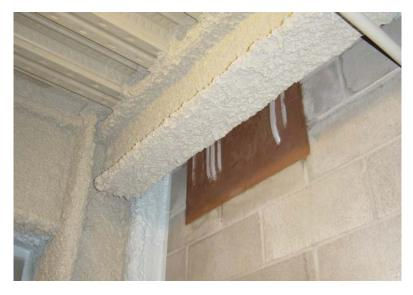
Compartmentation and structural protection make up part of balanced design with detection and alarms, sprinklers and occupant education. (Photos courtesy of Specialty Firestop Systems Inc.)
