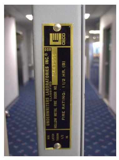
Fire resistance rated doors and hardware provide continuity to compartmentation. (Photo courtesy of Door & Hardware Institute)
