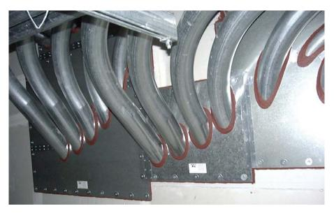
Compartmentation is completed when holes for condiuts are sealed effectively to maintain the fire resistance rating of the wall. (Photos courtesy of Specialty Firestop Systems, Inc.)
