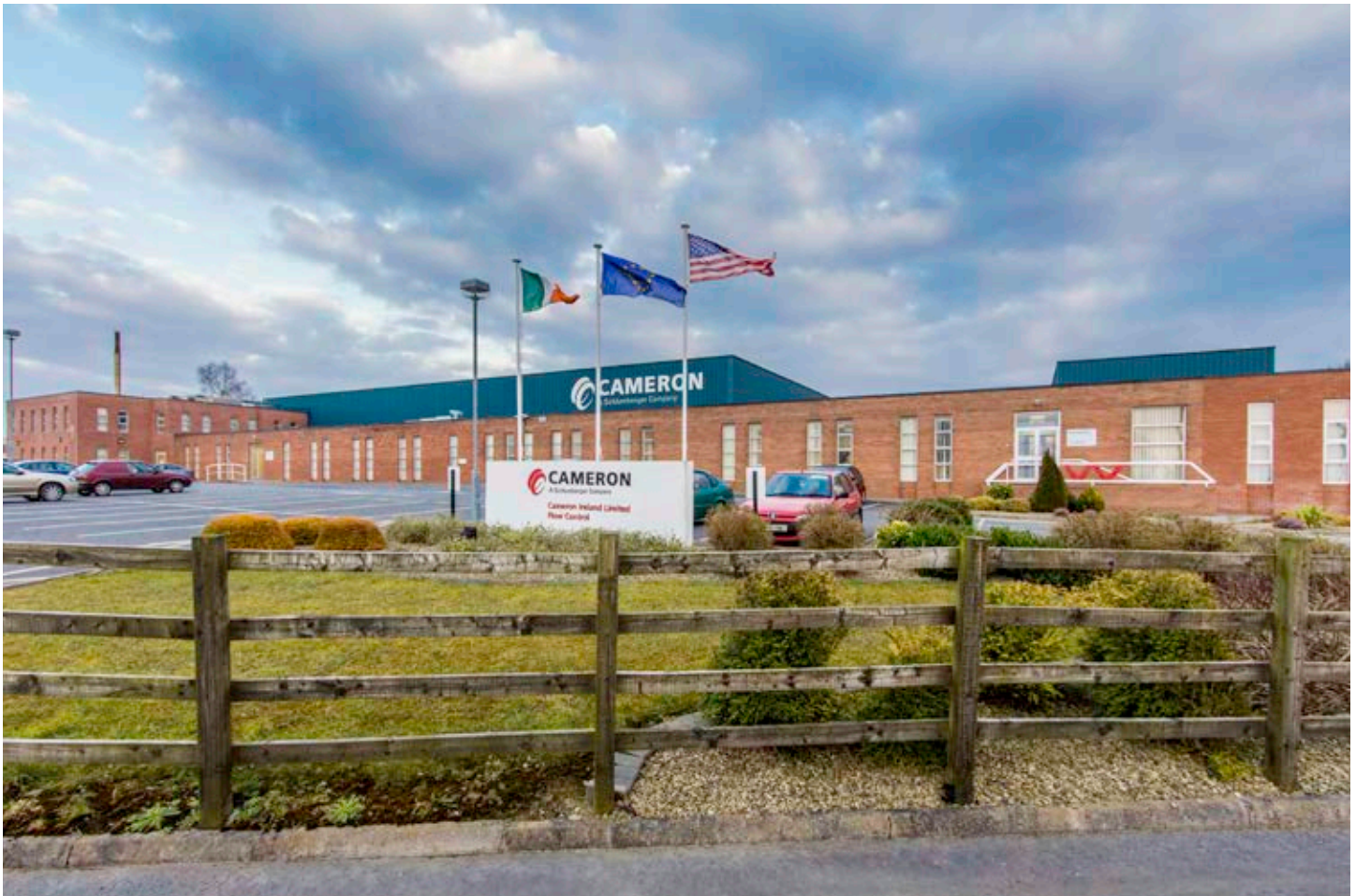
Cameron PULSE CIMV and subsea choke facility in Longford, Ireland.
