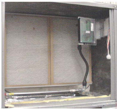
Fig. 22 - Return Air Sensor Operating Position
