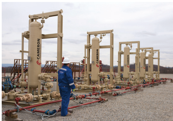
Cameron sand separators minimize solids in flowback fluids and production streams.
