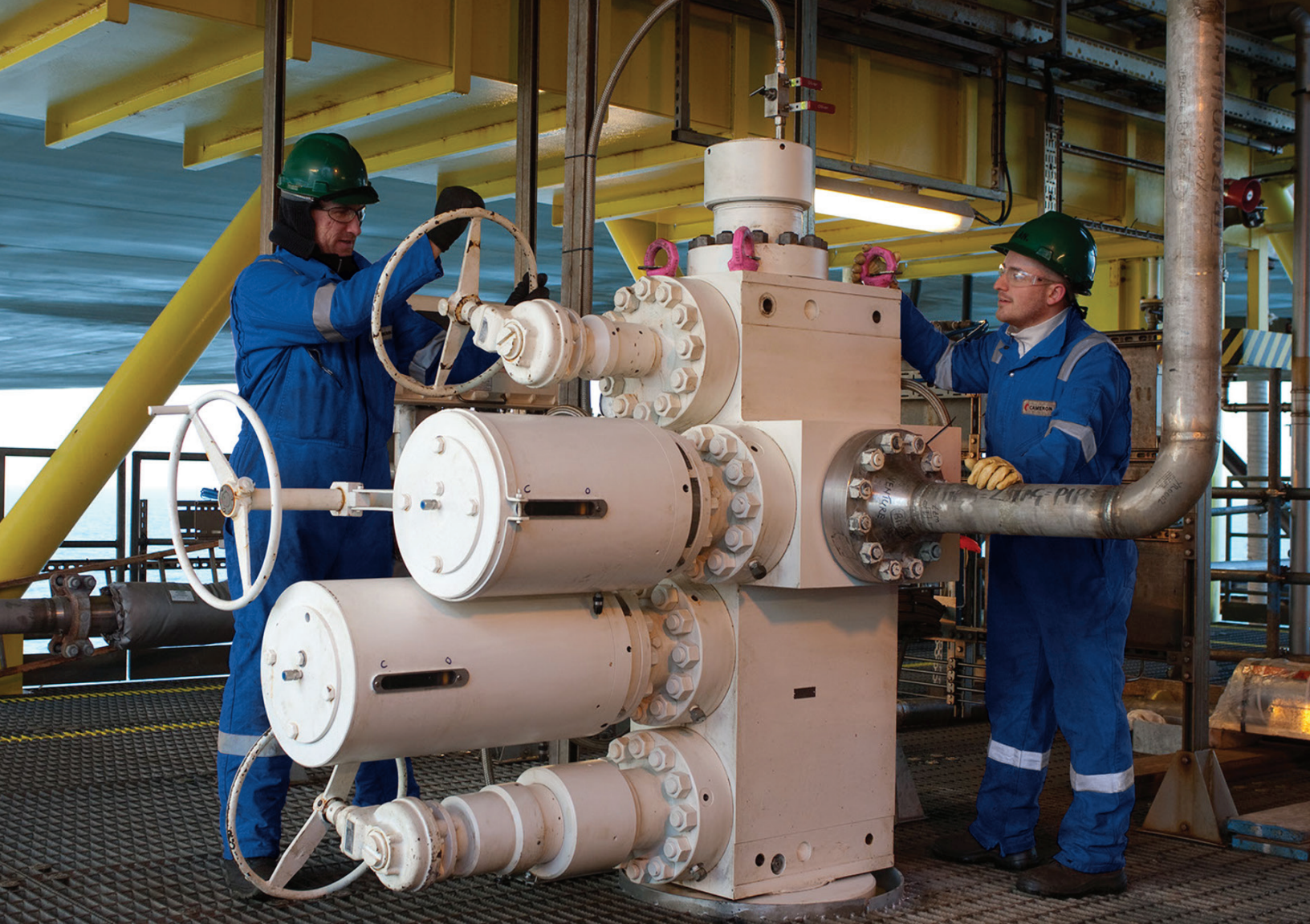
A team of experienced Cameron technicians performs all installations.
