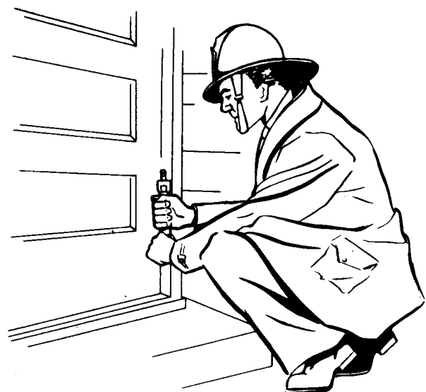
Figure 4-51. Removing the hinge pins.
