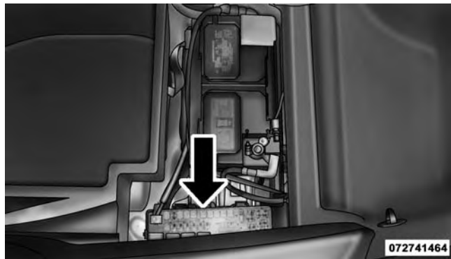
Rear Power Distribution Center
