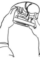
11 Using the pre-installed screws on the speaker, screw the speaker into the ceiling. Tighten the screws evenly until the speaker is flat against the ceiling.
