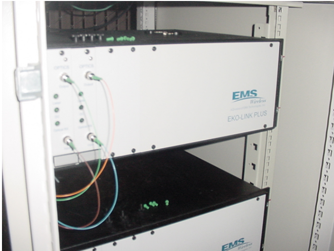
Figure 4: Rack Mounted EkoLink Plus Hub
