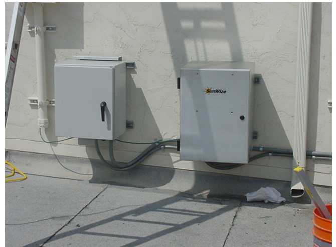
Figure 7: Remote Unit with optional Battery Back-up Unit
