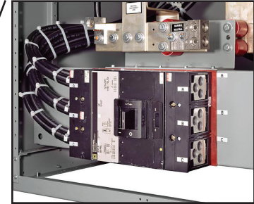
Fig. 13: Ground and neutral disconnect links
