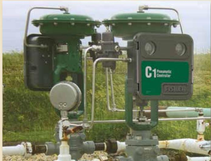
High consumption of compressed air or natural gas by instruments means high energy costs for plants.
