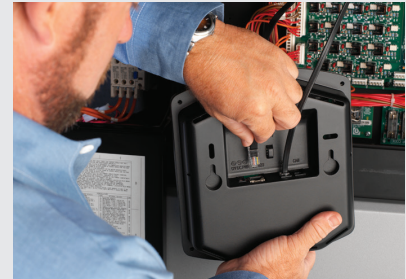
Removable display makes troubleshooting servicing easier.
