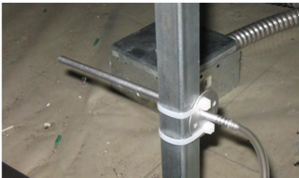
Figure 59 Static pressure sensor placement
