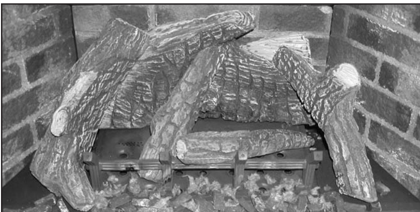
Figure 35. Fifth Stage Log Set Installation.
