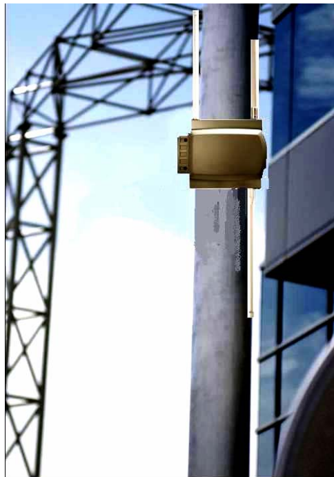
Fig 4. Typical BA100T with B2CG085AA module and antennas pole mounting arrangements
