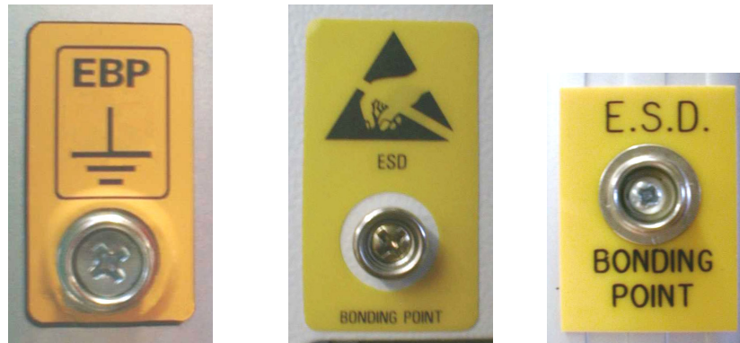
Fig. 3-1: Layout of Markings for Earth Bonding Points (Examples)
