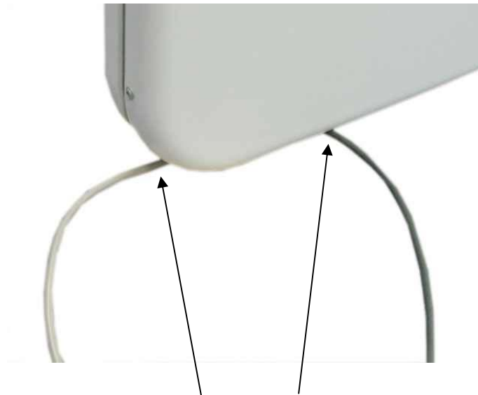
Fig. 5 Cable routing at the antenna sides
