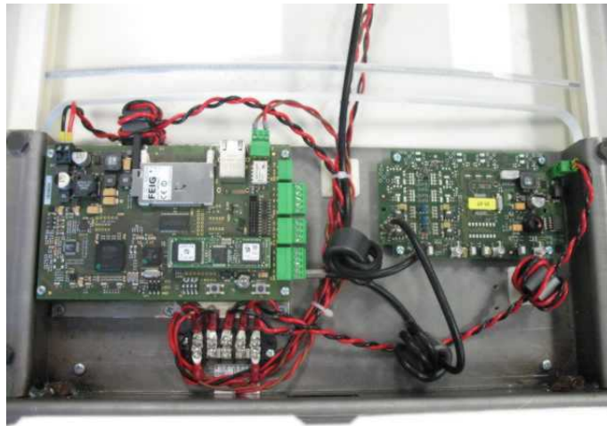
Fig. 10:Tying the cables
