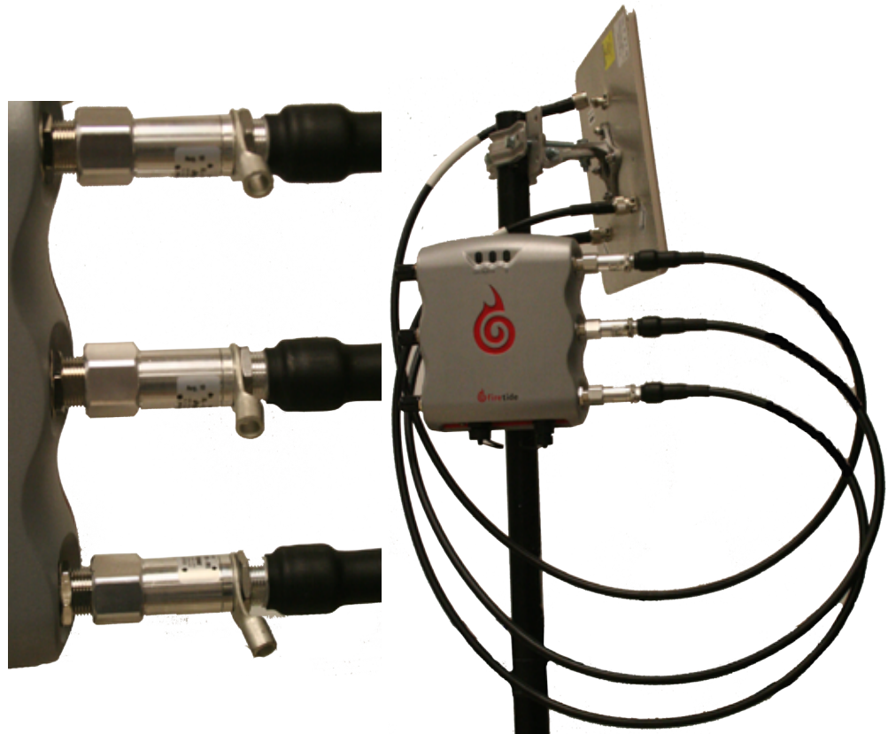
Figure 7. Cable-to-Radio Connections; Completed Installation
