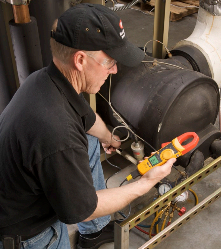
Liquid line temperature measurements for subcooling.
