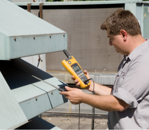
Taking measurements at the intake of a rooftop unit.
