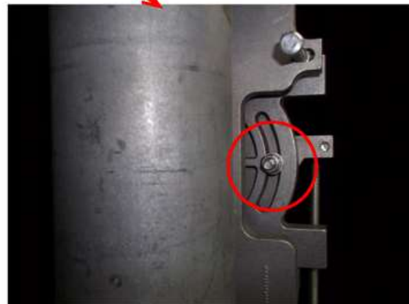
Elevation Fixing Bolt (Antenna rear side)
