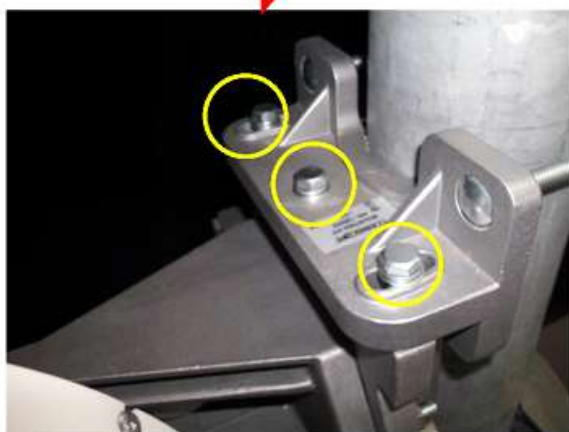
Azimuth Fixing Bolt (Antenna upper side)
