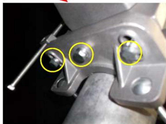
Azimuth Fixing Bolt (Antenna lower side)
