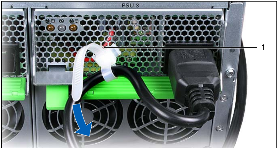
Figure 10: Using cable ties
