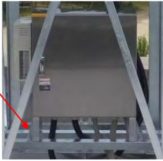
1. Fix the storage box on the ground or fixed steel using M10 bolt x4pcs.
