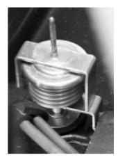
the bottom, or base pan, of the unit. When the plug is blocking the hole, as it should be during cooling operation, the condensate water is contained in the base pan. At temperatures when heating is required, the bellows contracts, the rubber plug is retracted from the hole and the heat pump condensate water is allowed to drain into the wall case. The valve is fully open at 49°F.
