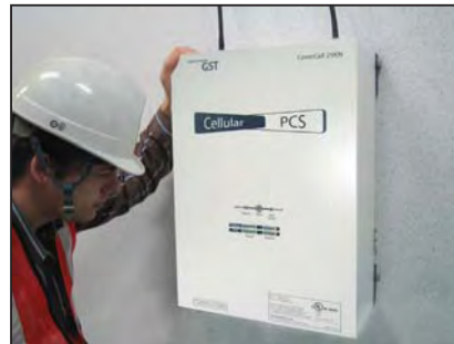
<Figure 10> Verification of LED Lights
