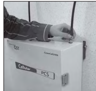
<Figure 7> Coverage ANT Port Connection
