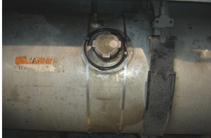
Figure 71: Installation with Metal Strips
