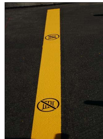
Finished Perimeter Stripe
