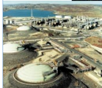
Woodside - Australia MS5002C LNG main refrigerant compressor drive
