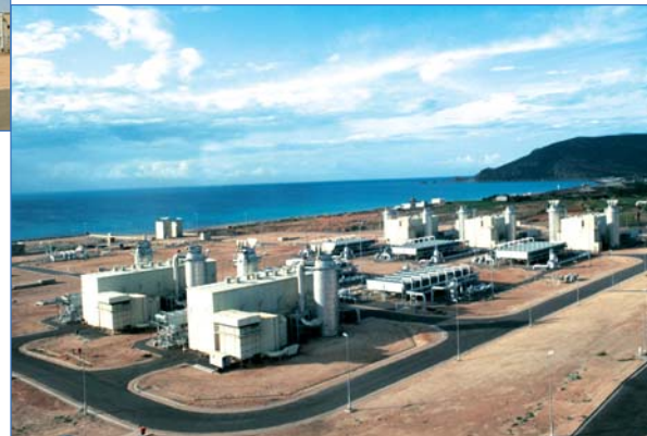
Cape Bon - Tunisia Trans-Med Pipeline Cape Bon to Sicily Head Station 25 MW Gas Turbine Driven Booster Compressors. MS5002 - BCL404/a
