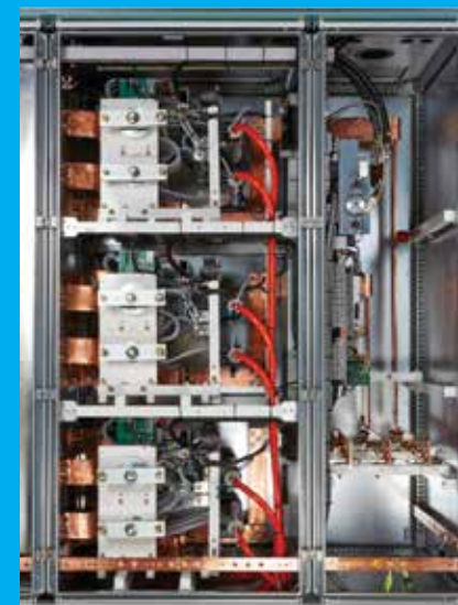
Inverter cubicle
