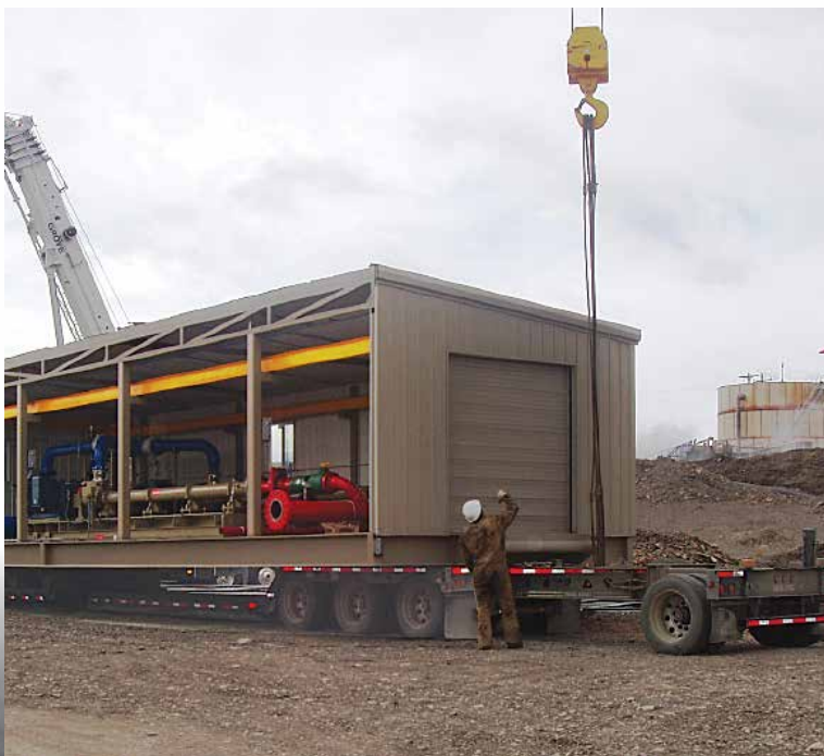
One-half of a custom fabricated skid-mounted enclosure delivered to installation site
