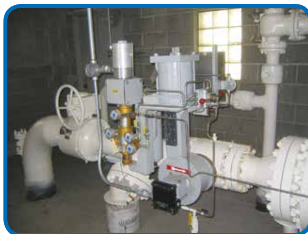
Figure 2 - Becker RPDA Actuated Control Valves
