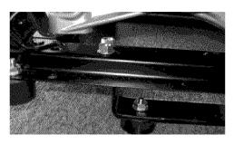
3) Thread the nuts onto the bolts.
