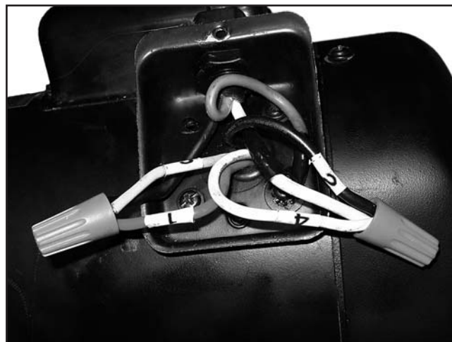
Figure 62. 110V motor wiring.
