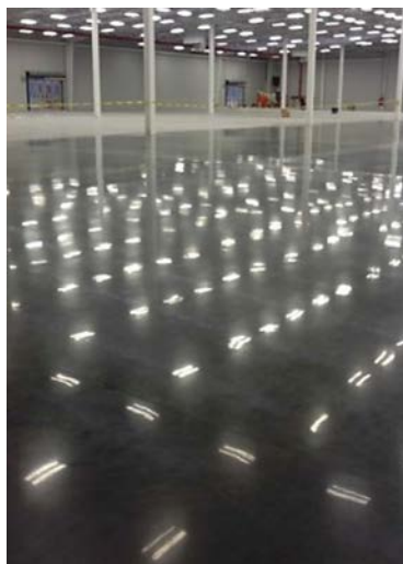
Concrete Polishing at its best!
