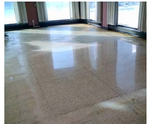
Marble Floor Restoration using the STI MG2 Diamond System and the P/M Machine
