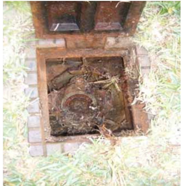
2. Clean the Hydrant or Valve with a wire brush
