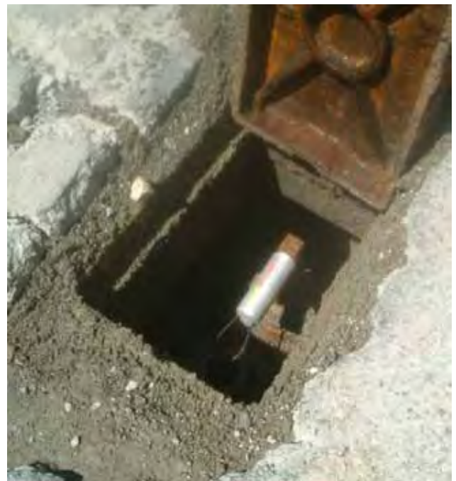
3. Make sure there is a good, clean, magnetic contact to the valve stem or hydrant. For optimum sound and radio transmission deploy the Zonescan vertically. To prevent the Antenna touching the metal lid and reducing transmission, fit a polystyrene block between the lid and Antenna.
