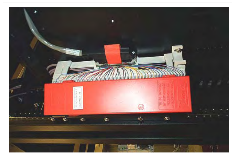
Figure 3-11: DPS Alarm Punchblock Connector
