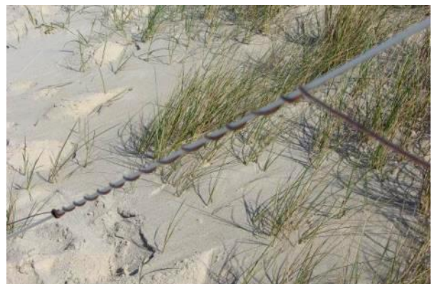
Radials twisted around guide rope
