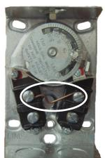
stops. A good initial setting for this pointer is 100 to 110 degrees. If it is set too low, the air will feel cool coming out of the registers at the end of the blower cycle.
