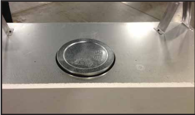
Figure 9.1 Seal Cap in Position
