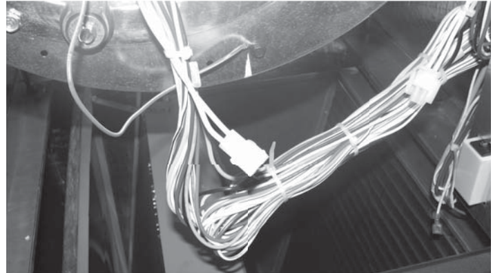
Figure 9: Install Two Pin Jumper Plug
