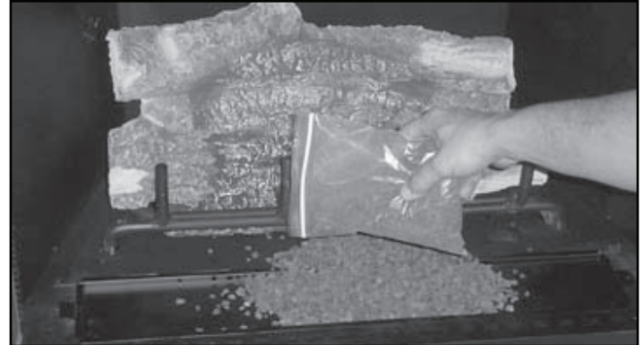
Figure 12.1 Placement of Lava Rock
