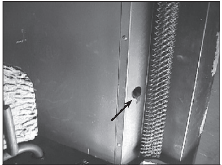
Figure 7.1 Outside Air Kit Handle Location
