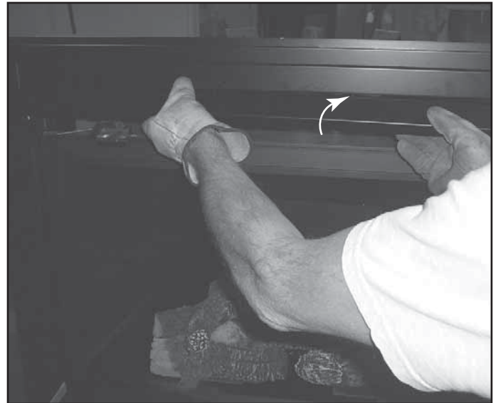
Figure 15.16 Intalling Hood
