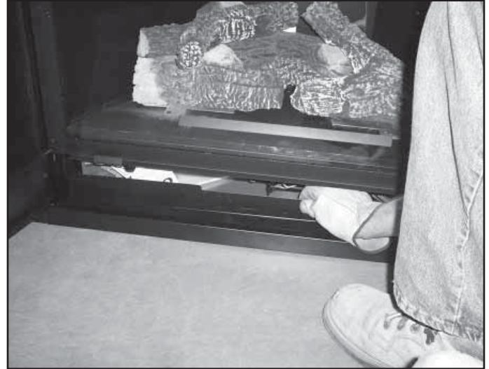
Figure 15.20 Installing Floor Cover
