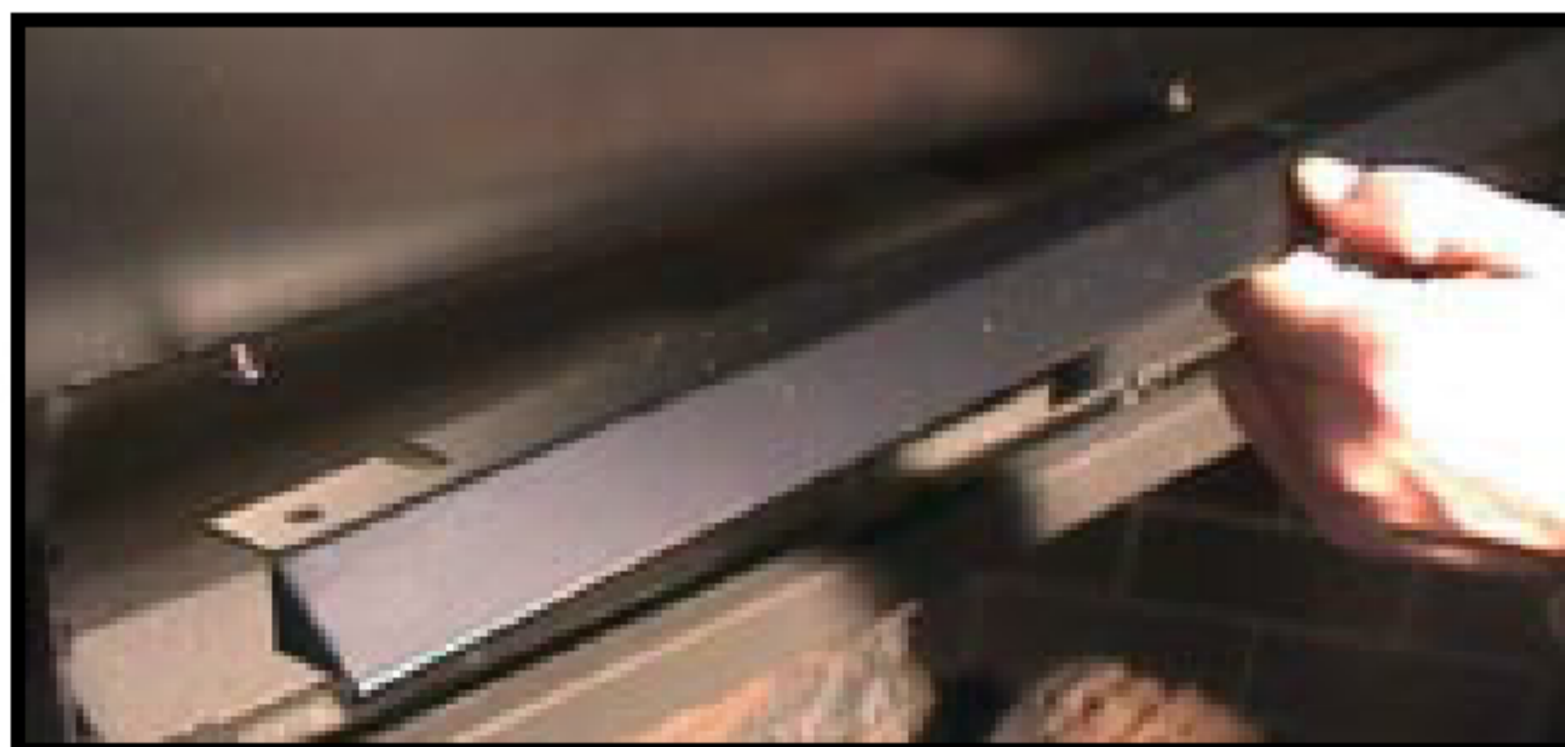
Figure 43 - Installing the Hood
