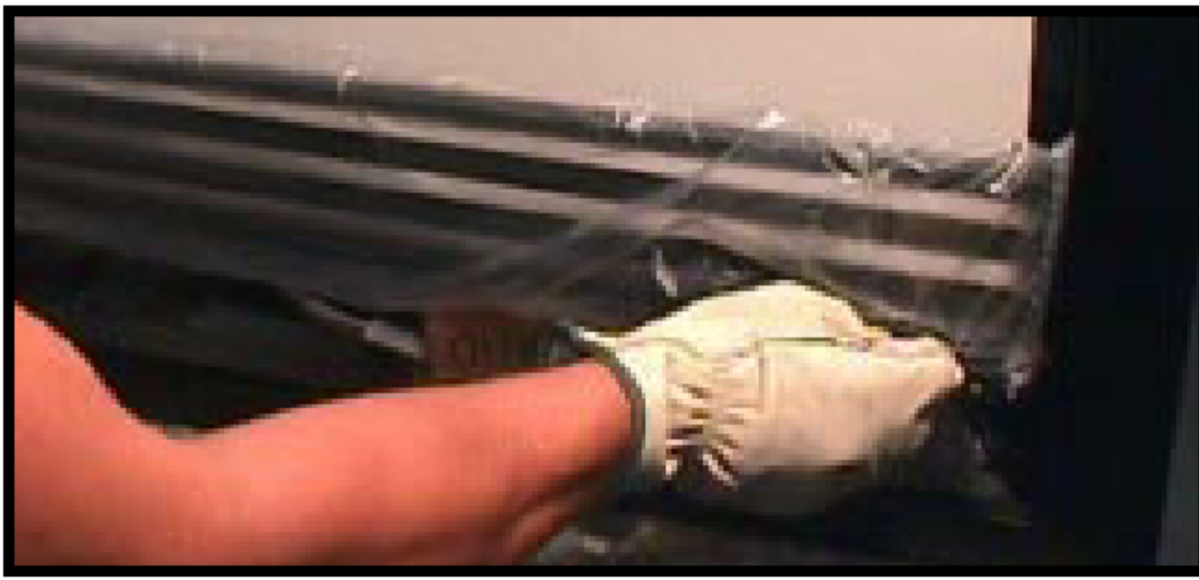
Figure 45 - Control Access Panel Removal
